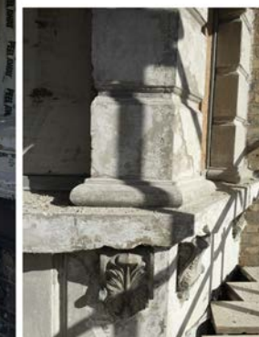
Fig 5.4. Photo 2017, during construction. The condition of the render and mouldings before repair work was carried out by specialist sub-contractor.
