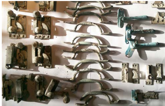
Fig 6.5. I asked the contractor to carefully dismantle all ironmongery to see what could be cleaned, what is still forged / made in similar manner. [d]
