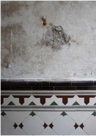
Fig 6.1. Pre-strip out condition of lime plastered brick internal wall with C19th tiling mostly intact.
