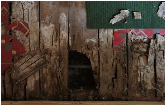
Fig 6.3. The floor of the south east corner of room 1.04 had clear evidence of fungal rot, caused originally by unattended leaking gutter. [f]
