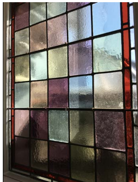
Fig 10.2. Window W1.01A. Stained glass leaded lights restored by local specialist sub-contractor Rob Croudace.
