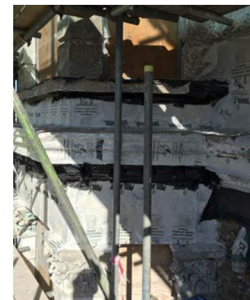
Fig 5.3. Photo 2017, during construction. Paint being stripped from the render and mouldings with a poultice.
