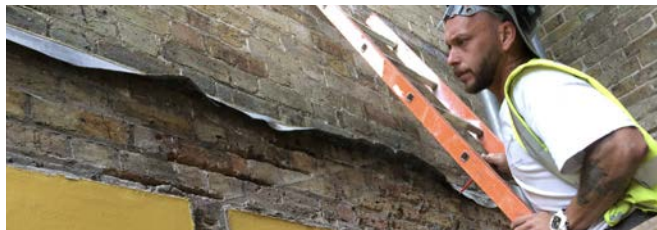
Fig 9.6. Foreperson Simon Aspinall inspecting the existing flashings during demolition, assessing suitability for re-use in same position. Also note scar of historic sloping roof, preceding the flat roof as found in 2015.
