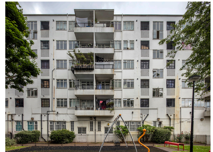
Full west elevation view
