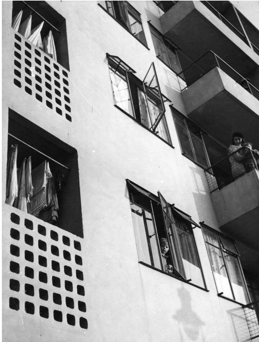
Kensal House. East Block, West Facade. Photograph by Edith Tudor Hart, 1937 (RIBA Collections).
