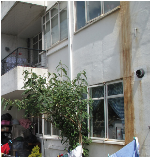
Site Photograph, 2019 The surface of the concrete is visible in the raking sunlight. You can discern the individual shuttering panels, and the smooth surface under the paintwork.
