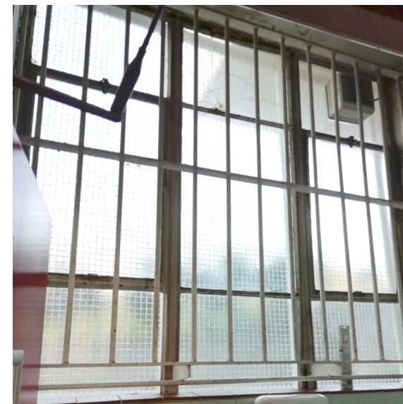
Photo of original window in Western Block
